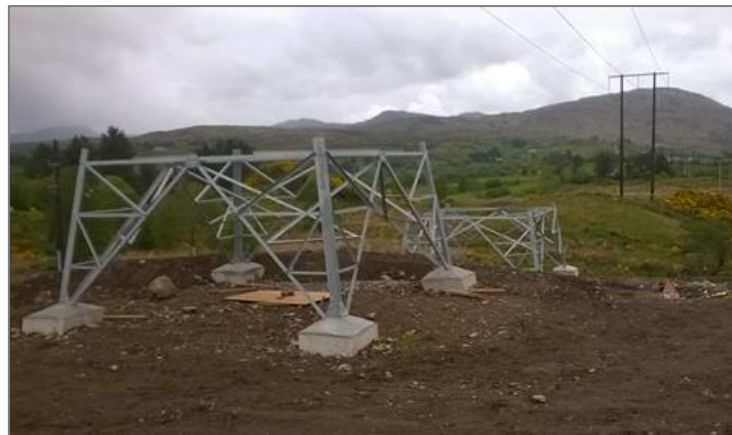
Figure 14 - 110kV Interface Mast Foundation Complete
