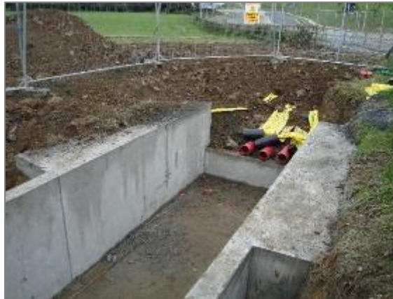
Figure 9 - Completed joint bay prior to cable installation (in-situ)
