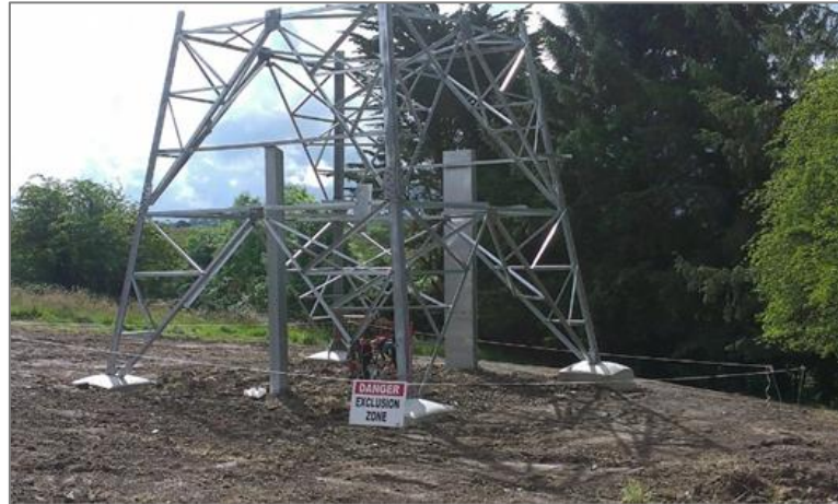
Figure 15 - Base of Interface Mast Structure Backfilled
