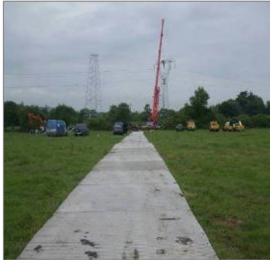
Figure 17 - Temporary Aluminium Panel Tracks
