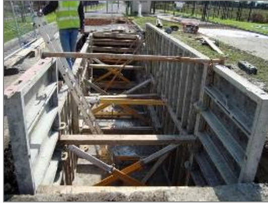
Figure 8 - Typical joint bay under construction (in-situ)
