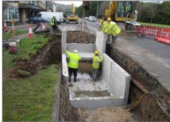
Figure 10 - Typical joint bay under construction (pre-cast)
