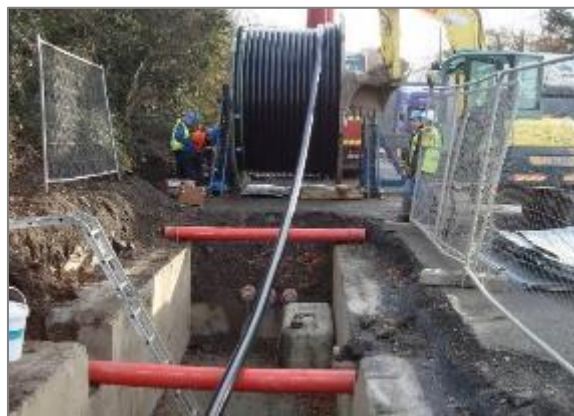
Figure 11 - HV cable pulling procedure (Typical drum set-up)
