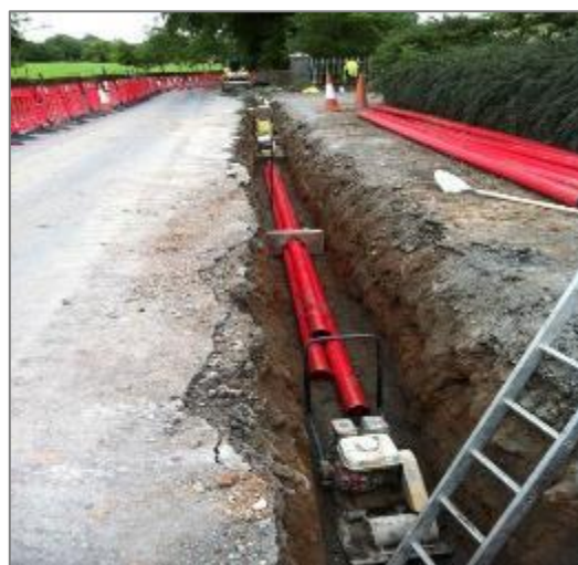
Figure 2 - Typical 110kV Underground Duct Installation
