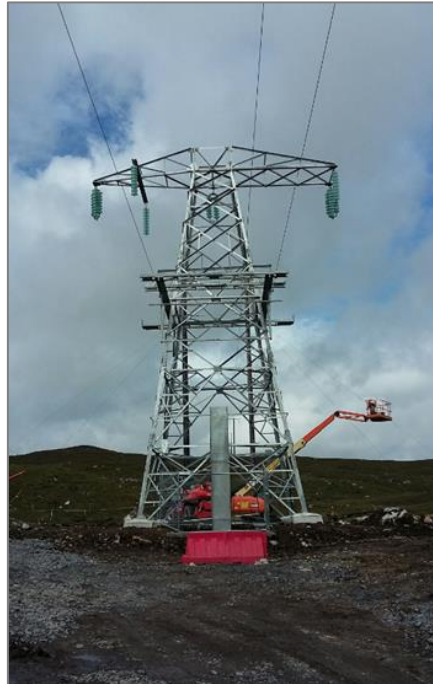
Figure 16 - Completed Line/Cable Interface Mast
